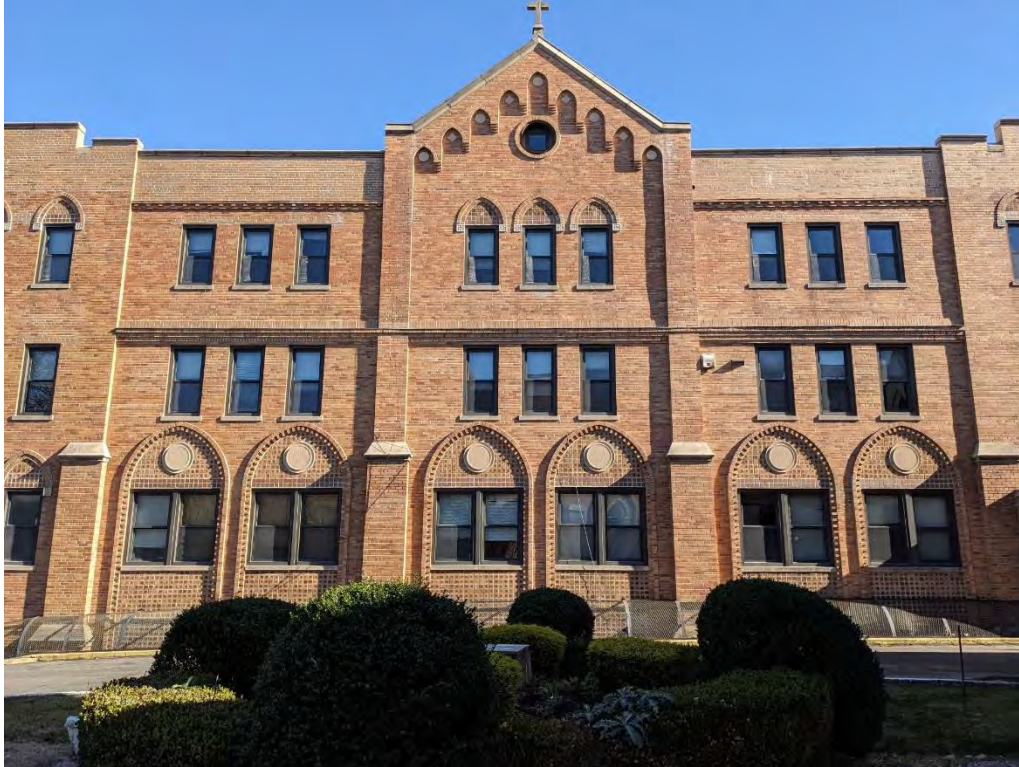
Photograph 5. The former elementary school building. View looking northeast.
