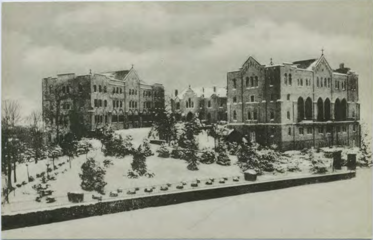
An undated view of the campus after the third story had been added to the elementary school and the chapel had been constructed, looking southeast.
