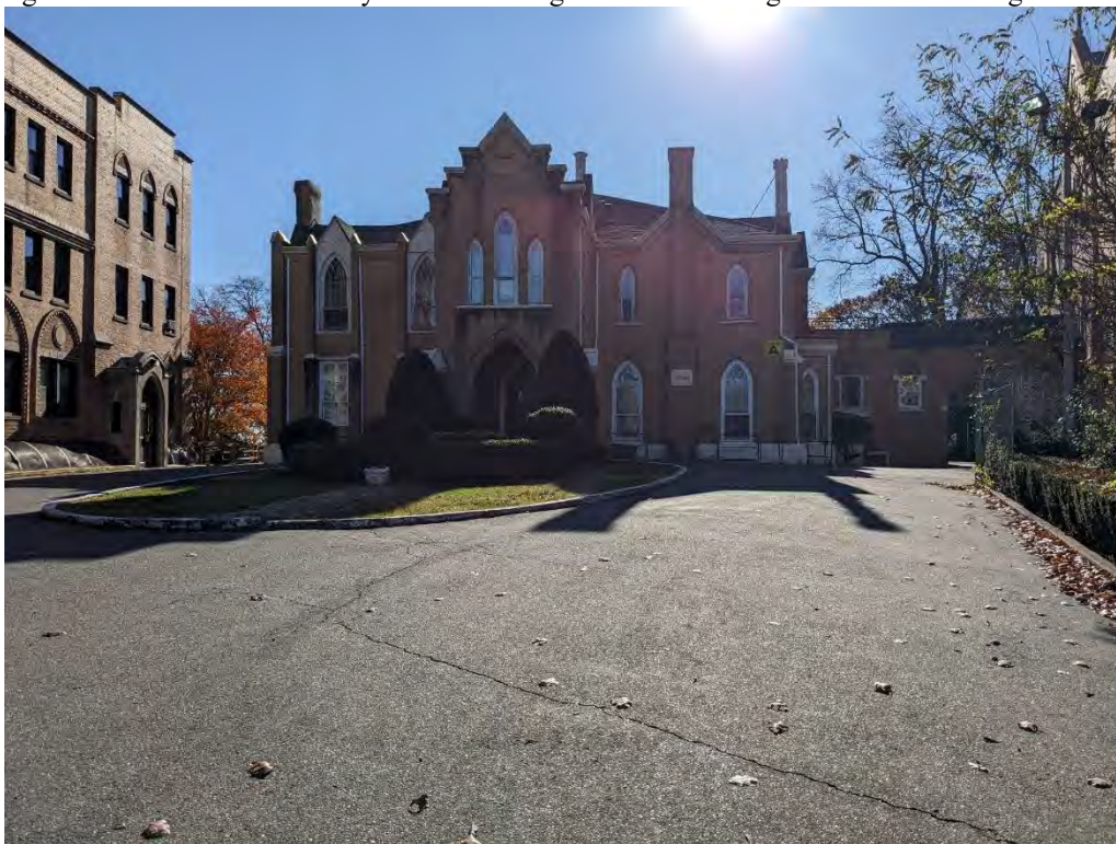
Photograph 2. The former Villa building, flanked by the former elementary school on the left and the former chapel on the right. View looking southeast.
