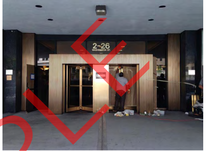
A.6: Southwest Entry Exterior (Main Entry)
