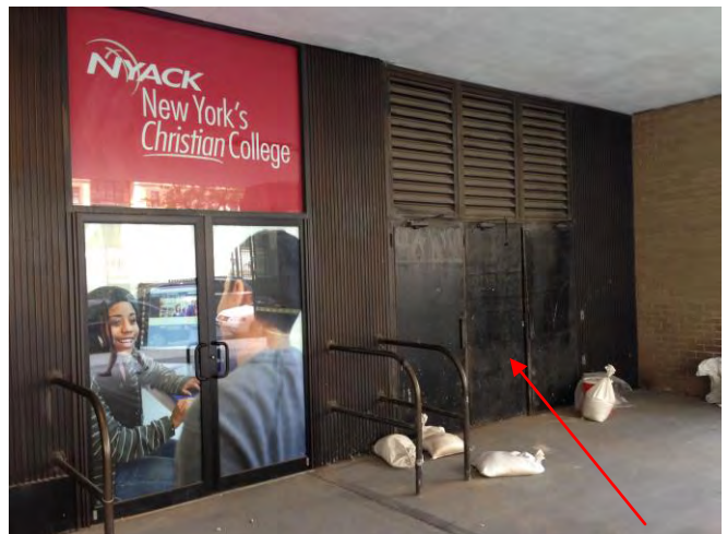
A.8: South Entry/Exit to 2 nd Fl. Roof
