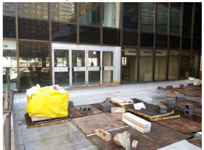
A.34: Re-entry Doors (to Second Floor)
