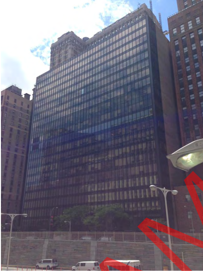
A.1: Southeast Façade
