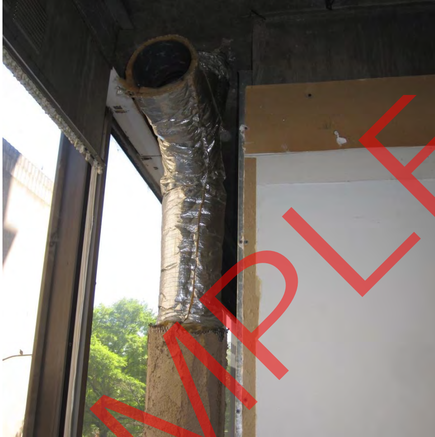
Photo M-6: Perimeter induction box air plenums and heating/cooling coils
