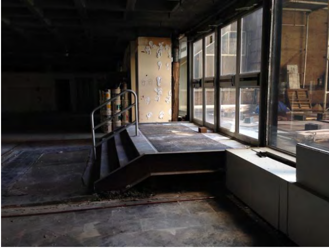
A.28: Doors and Stair to Roof Terrace
