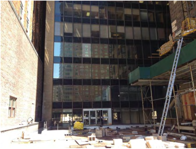
A.31: Roof Terrace (looking East)
