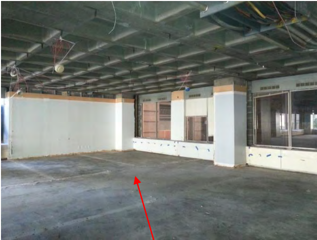
A.24: View Looking West
