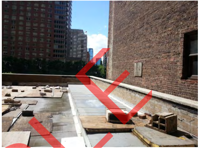
A.32: Roof Curb (looking West to Battery Park)
