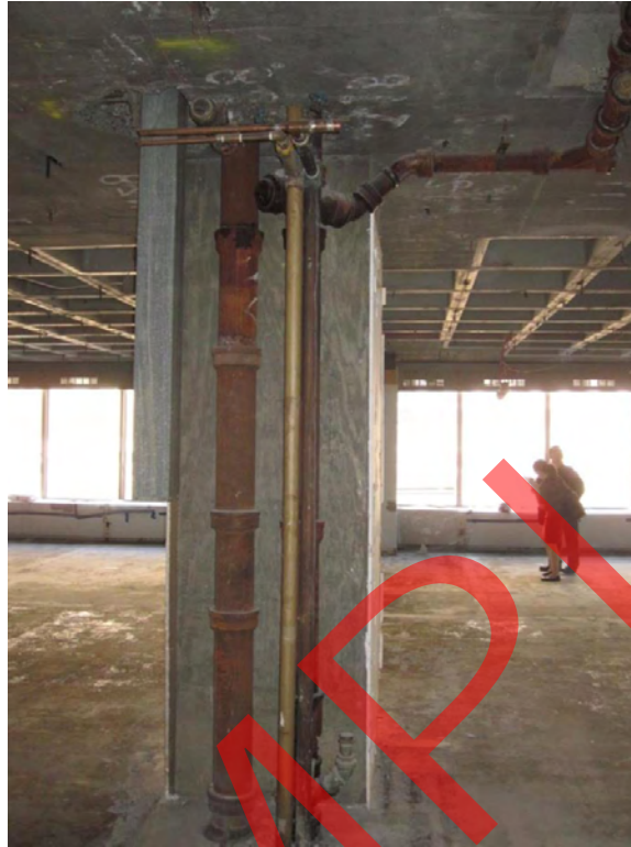
Photo P-2: Wet stack in 2 nd floor
