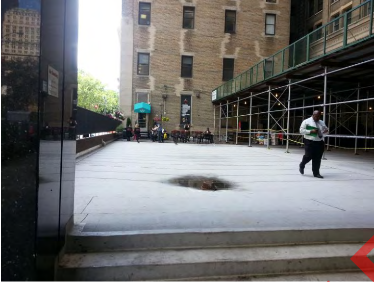
A.9: Adjacent Southwest Plaza
