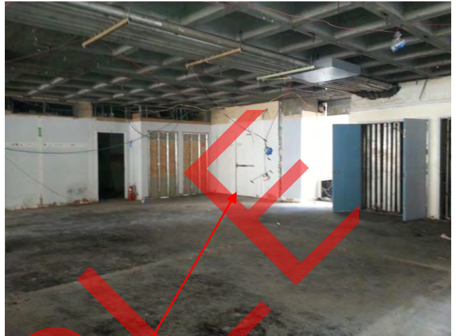
A.25: View Looking West (Passage to 17 Battery Pl.)
