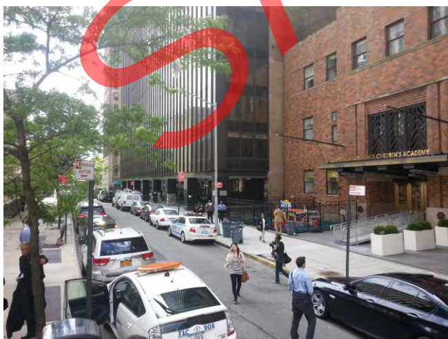
A.3: North Façade (at Washington Street)
