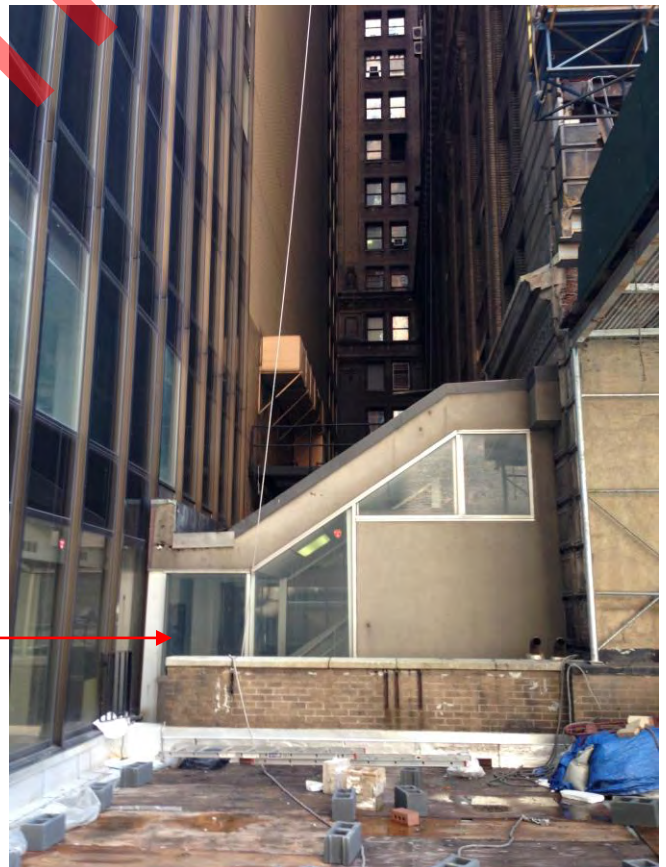
A.27: Passage to 17 Battery Place (Exterior)
