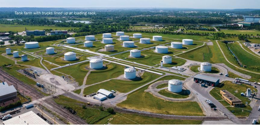
The type of roof is what makes the difference for most storage tanks. Some tanks are built with a solid cone roof with vents along the perimeter. Other tanks may only have a floating roof and some tanks may have an aluminum geodesic dome installed over a floating roof.
