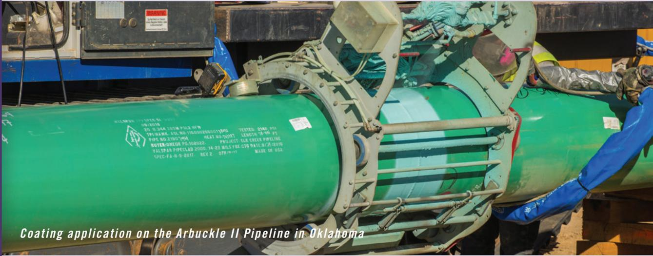
*Coating application on the Arbuckle II Pipeline in Oklahoma*
