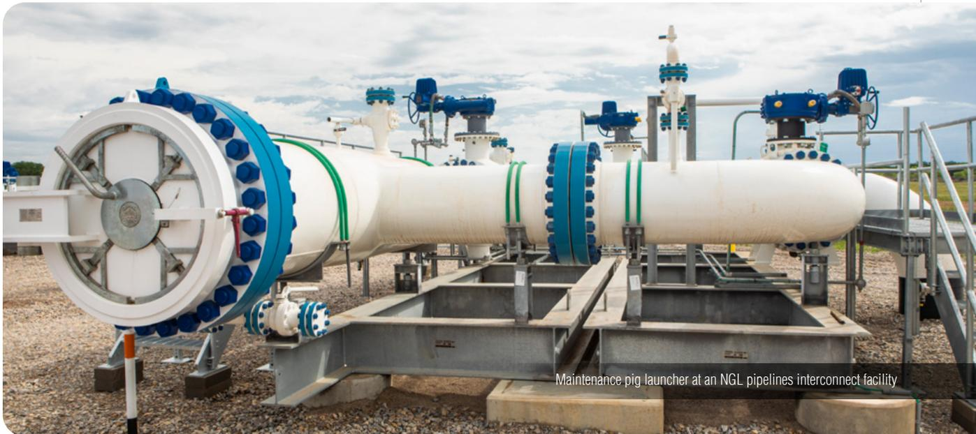
Maintenance pig launcher at an NGL pipelines interconnect facility
