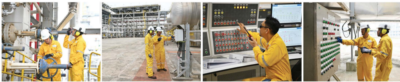
Crude heater firing by Area 1A team
