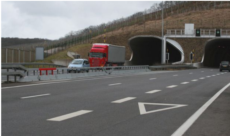
Left: Median barrier with colour-highlighted emergency gate
