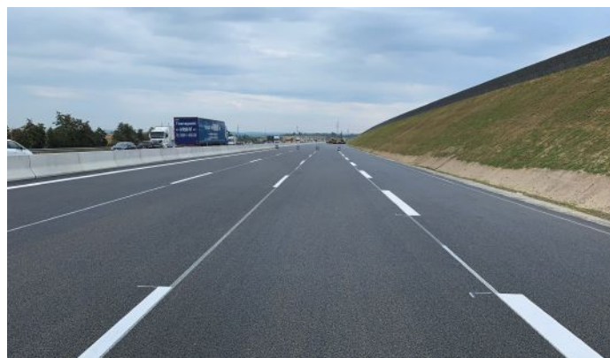
Above: The in-lay application of preformed tapes on new asphalt means roads can be opened for traffic quickly
