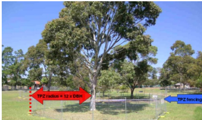
Figure 11: TPZ fencing is erected around retained trees prior to site works.
