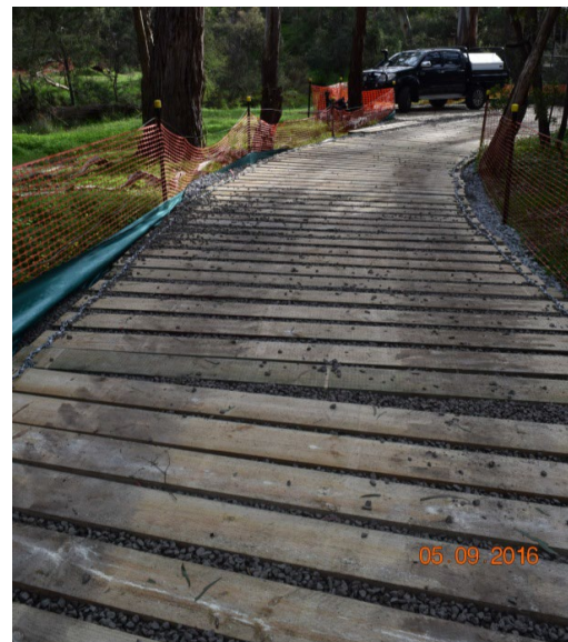
Figure 14: Rumble boards over crushed rock.
