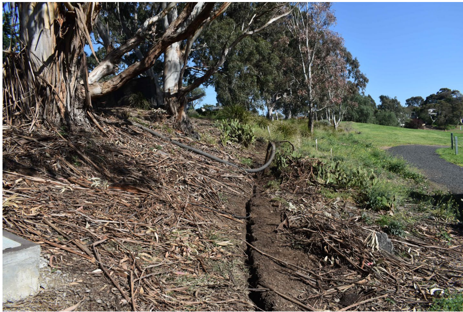
Figure 3: Trench adjacent Trees 6 and 7
