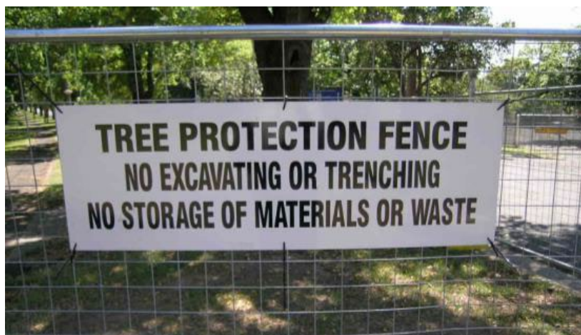
Figure 12: Example of a TPZ warning sign clearly displayed on TPZ fencing.
