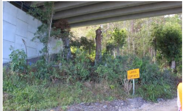
D) Extended bridge underpass adjacent to the Richmond River, showing tall stumps retained during construction for arboreal species, Pacific Hwy, NSW.
