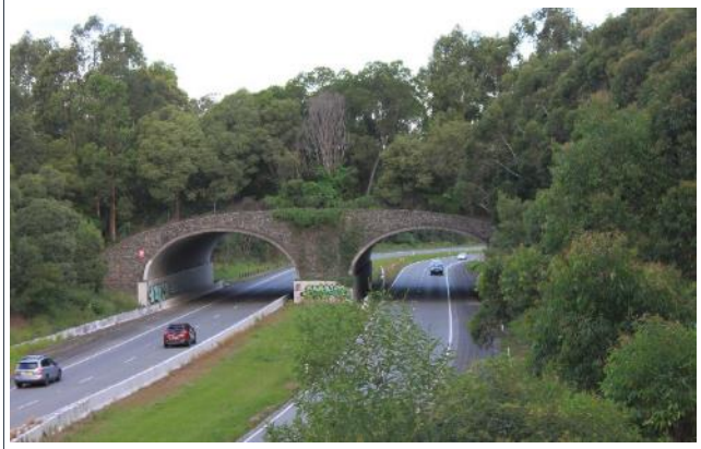
B) Land bridge over Pacific Hwy, Yelgun NSW.
