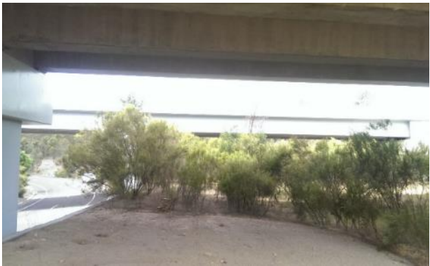
C) Extended bridge underpass adjacent to Metcalfe-Taradale Rd, Calder Freeway, Vic.
