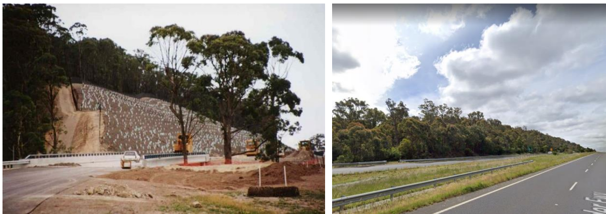
Figure 316. Example of large cutting (Calder Freeway) where significant benching, soil preparation, planting and mulching has been done. Immediate impact reduces over time through vegetation growth. Construction occurred in 2001 (left hand image) and is shown in 2019 (right hand image) after significant vegetation growth.
