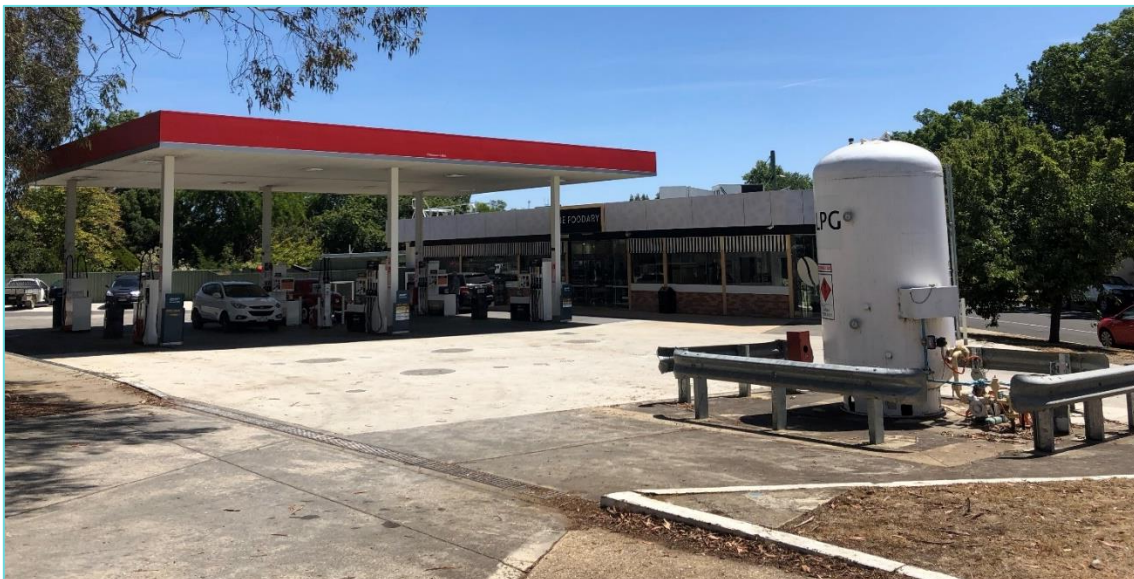
Figure 7.2: Caltex Service Station, Beaufort
