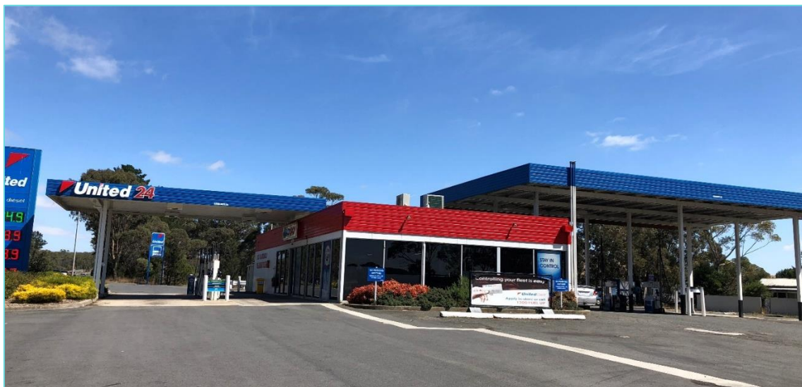
Figure 7.3: The United Petroleum Service Station, Beaufort
