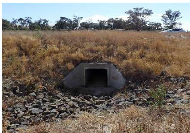
Photo 6.4 Box culvert at Western Highway
