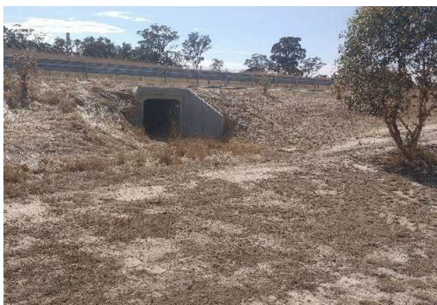
Photo 6.3 Box culvert located at slip road of west tie-in with Western Highway
