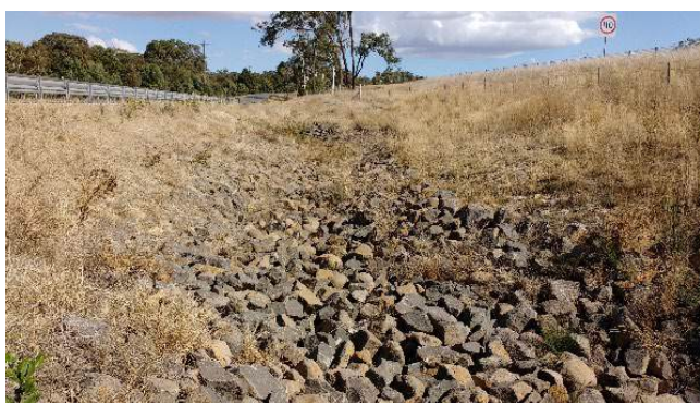
Photo 6.1 Rock lined channel located upstream of box culvert at Western Highway
