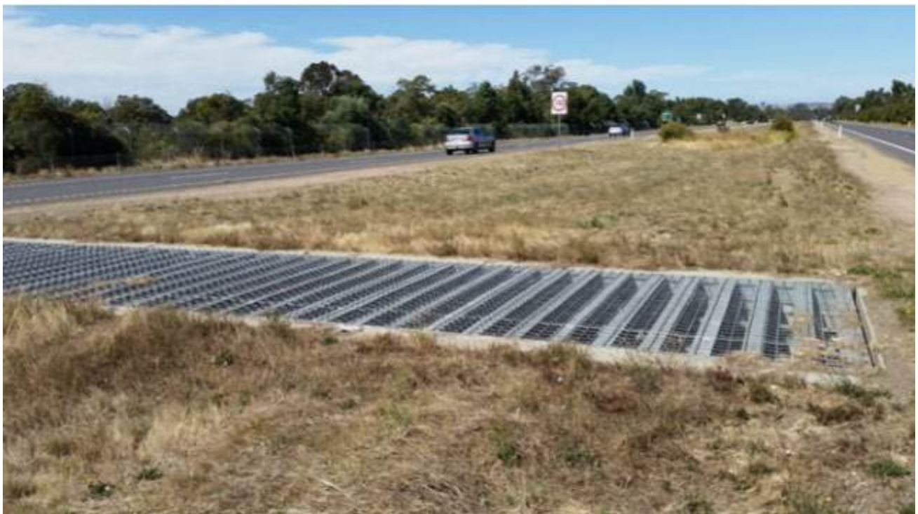
Photo 10.3 Example of light well in road culvert (source: Growling Grass Frog Crossing Design Standards, DELWP, 2017)
