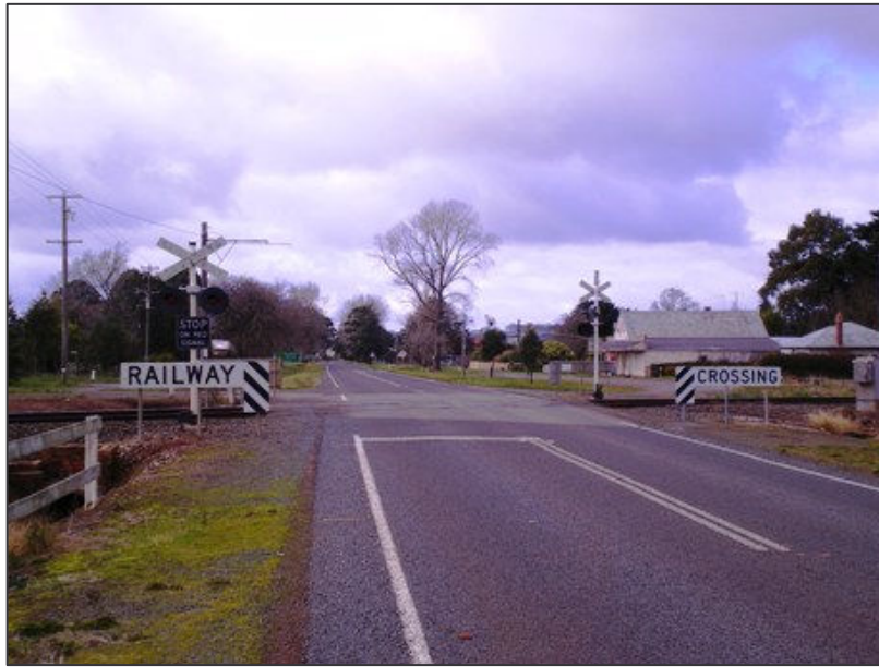
Figure A 3: Rail level crossing – Bungaree-Wallace Road in Wallace
