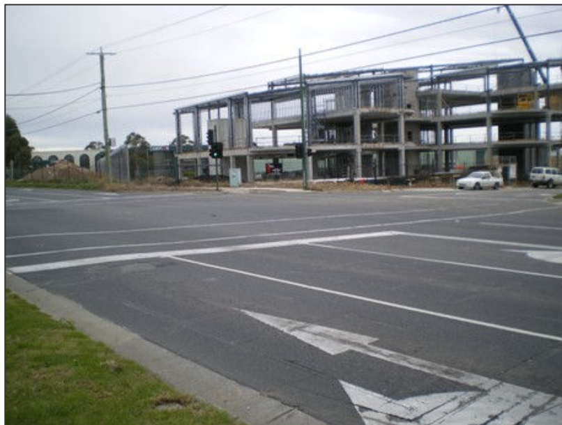
Figure A 12: Signalised intersection – Mitcham Road / Premier Avenue in Mitcham
