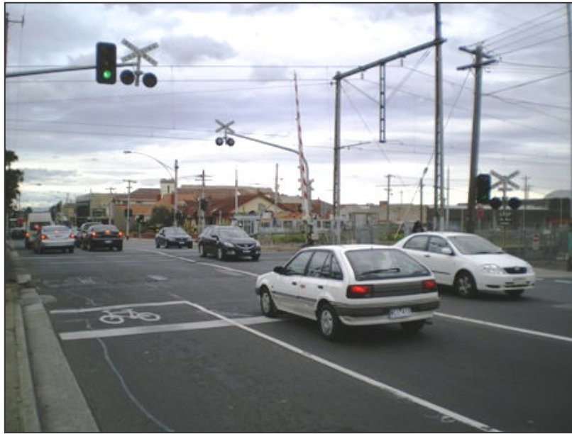
Figure A 11: Rail level crossing – Moreland Road in Moreland
