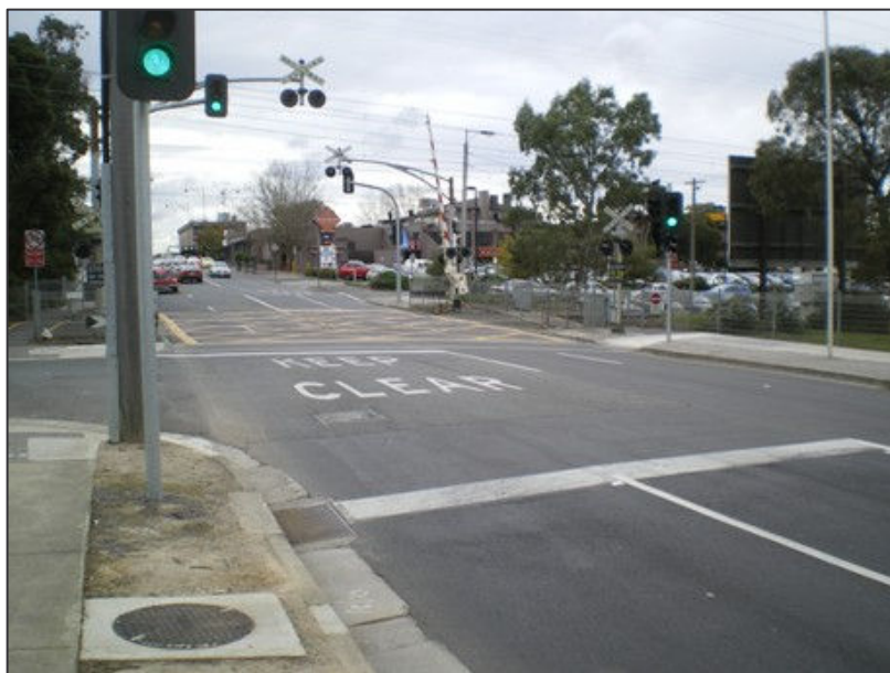
Figure A 10: Rail level crossing – Mitcham Road in Mitcham
