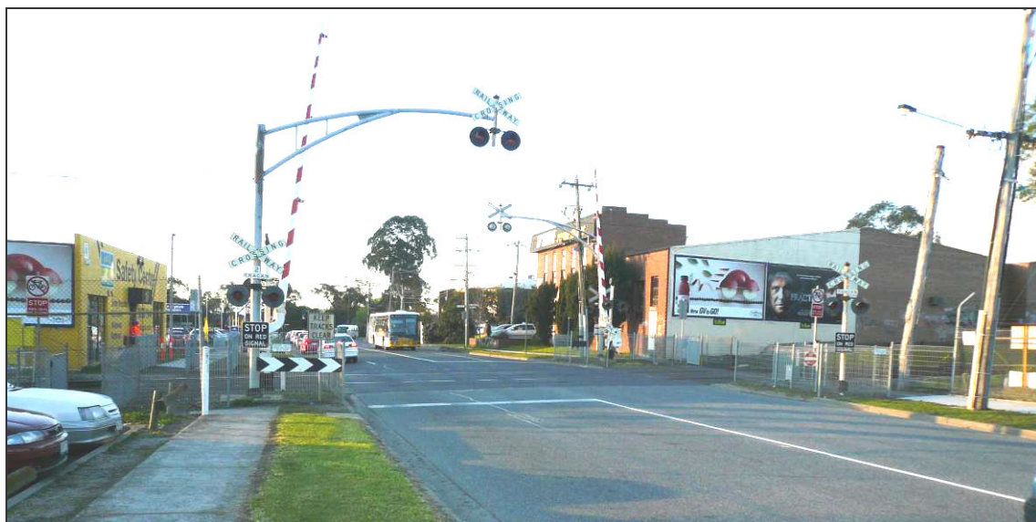
Figure A 6: Rail level crossing – Rooks Road in Nunawading
