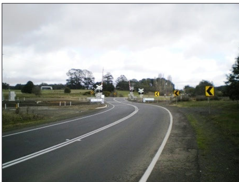
Figure A 8: Rail level crossing – Tylden-Woodend Road in Woodend
