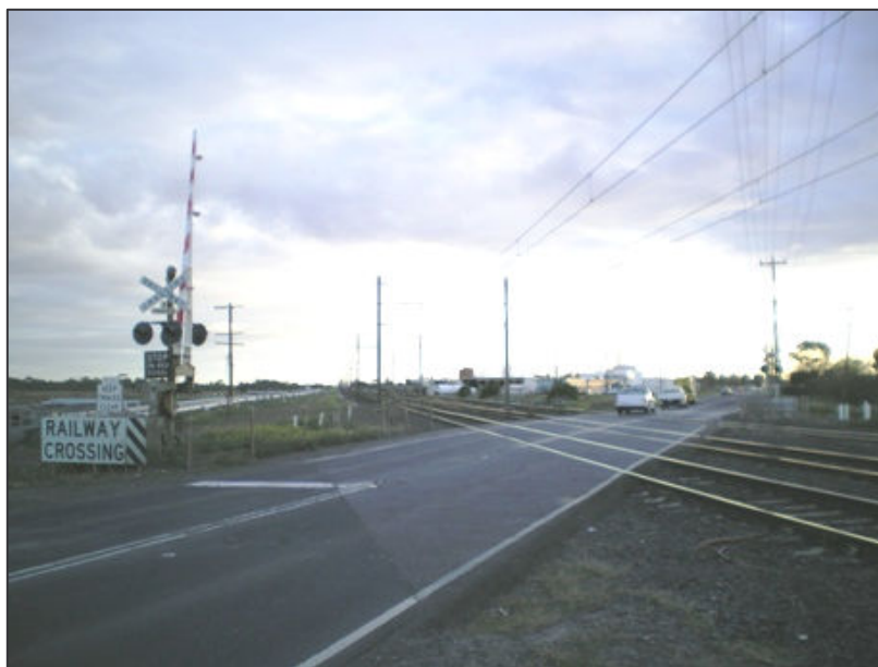
Figure A 9: Rail level crossing – Kororoit Creek Road in Altona
