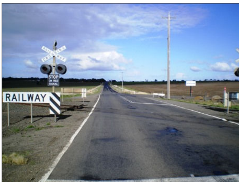
Figure A 5: Rail level crossing – Geelong-Ballan Road in Moorabool
