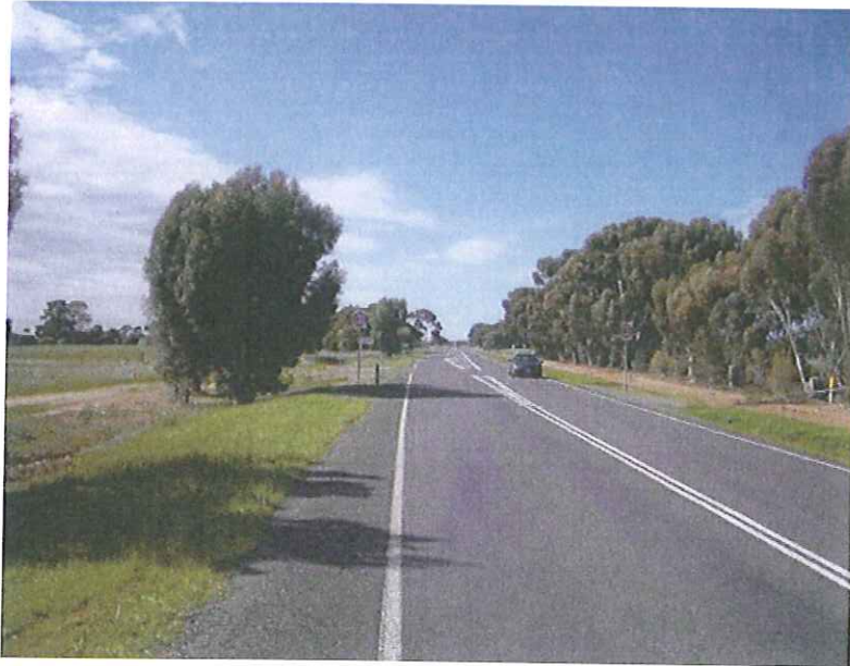
Figure B.1: Eastbound - approx 700 m from the level crossing
