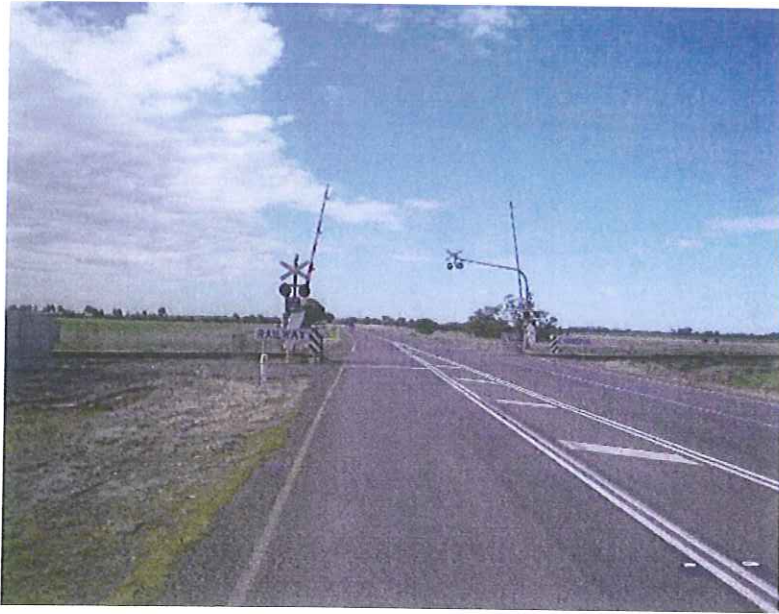
Figure B.3: Eastbound - at the level crossing
