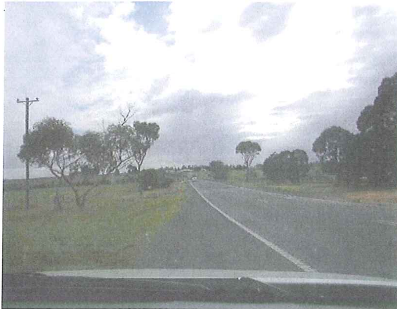
Figure A.1: Westbound - approx 800 m from the level crossing
