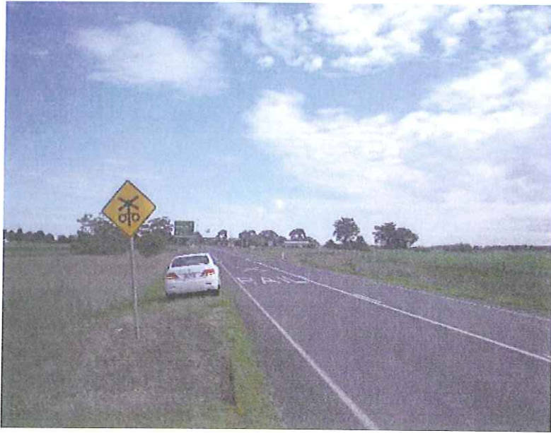
Figure B.5: Westbound - approx 200 m from level crossing
