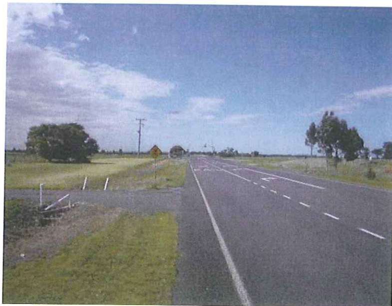
Figure B.2: Eastbound - approx 200 m from the level crossing
