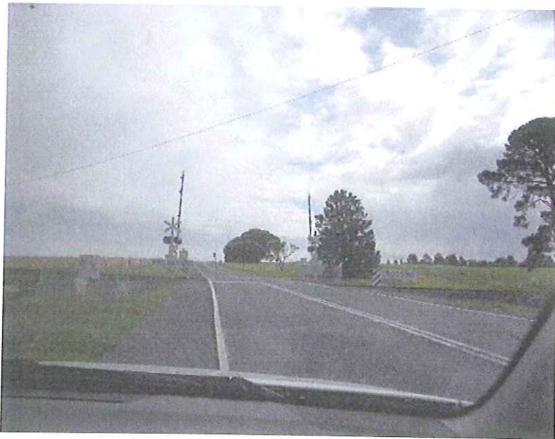
Figure A.3: Westbound - at the level crossing
