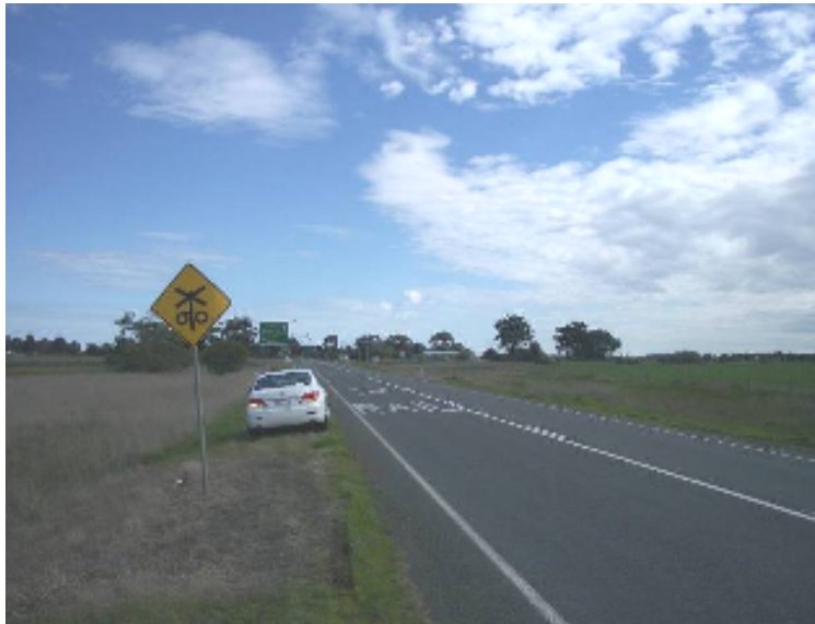
Figure A 5: Westbound - approx 200 m from level crossing
