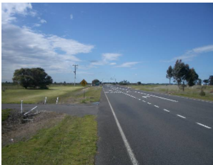
Figure A 2: Eastbound - approx 200 m from the level crossing
