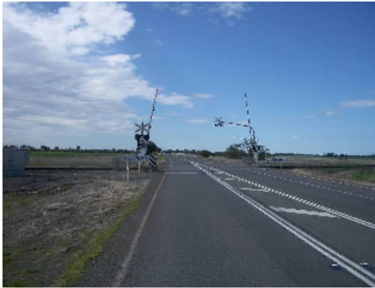
Figure A 3: Eastbound - at the level crossing
