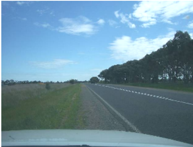
Figure A 4: Westbound - approx 800 m from the level crossing
