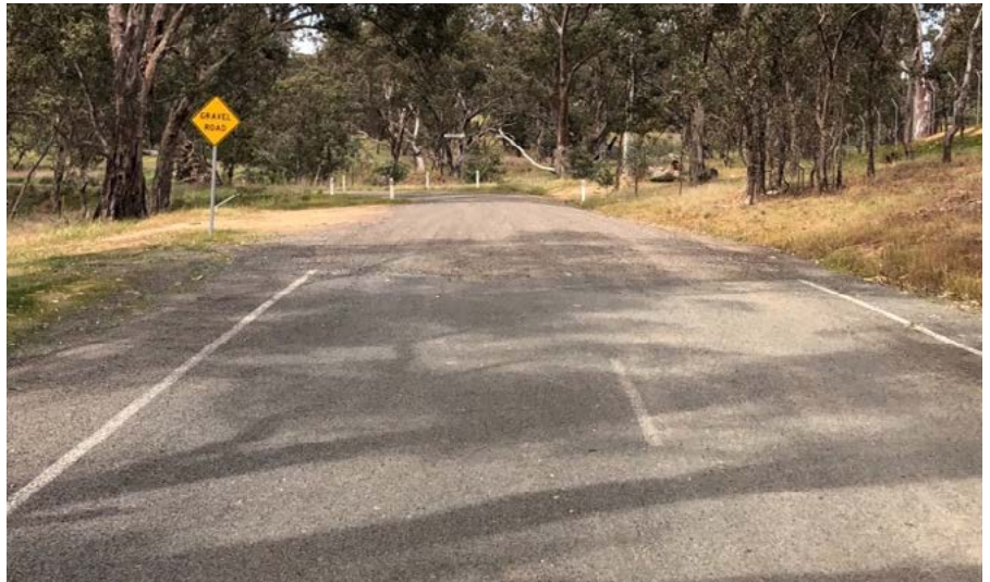
A change in surface type can result in a motorcycle losing traction, especially when one of the surfaces is loose gravel.
