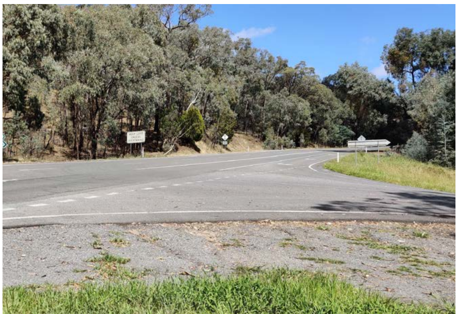
Sealed bell mouths can significantly reduce gravel carry-over.
