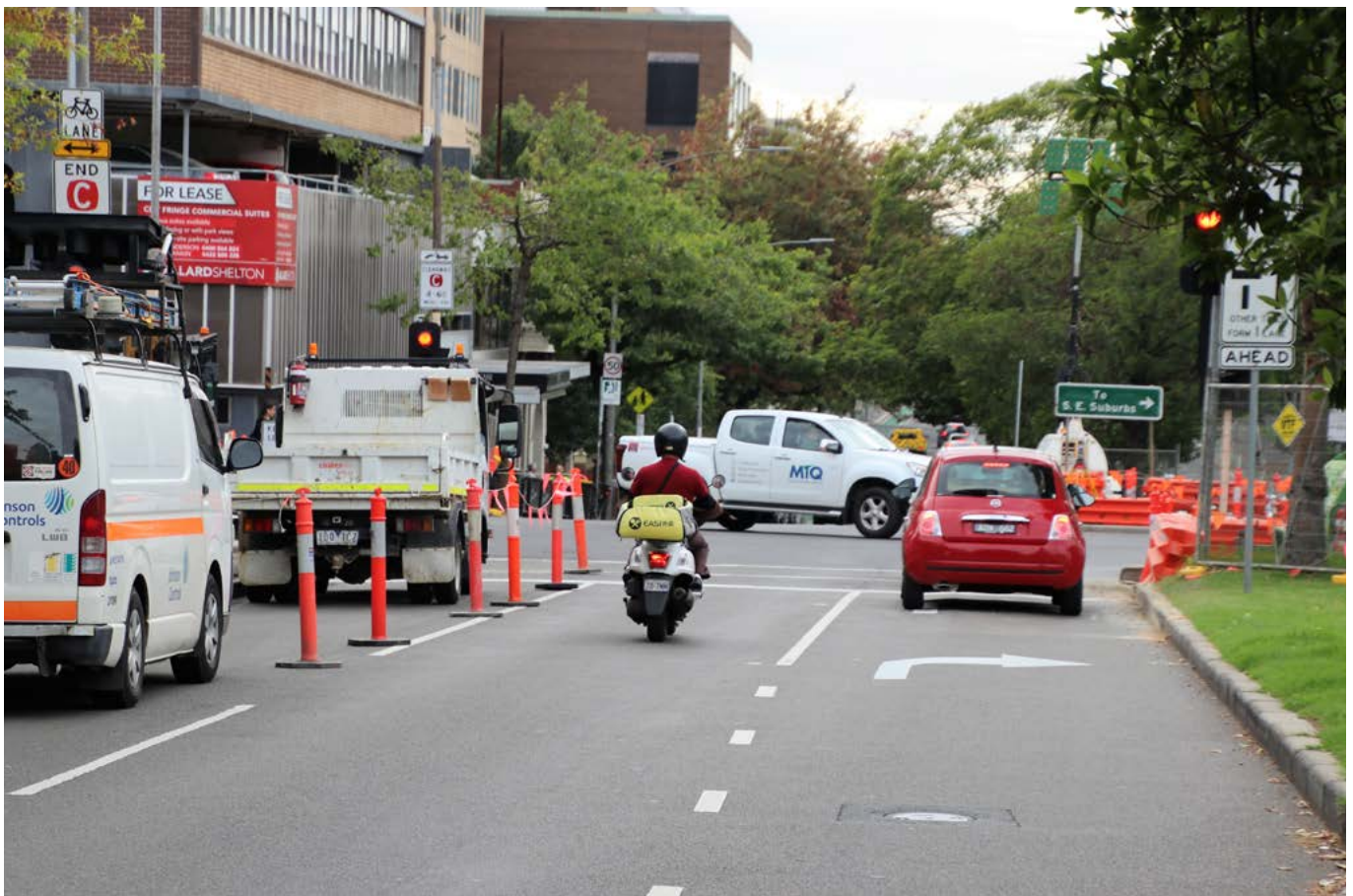
Road surface around construction zones should be kept clear of debris and the road surface should be kept leveled. Provide adequate warning of construction zones to road users by way of signage and lighting.
