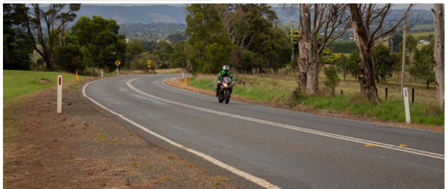
Delineators assist motorcyclists by indicating the direction of the road ahead, especially at night.
