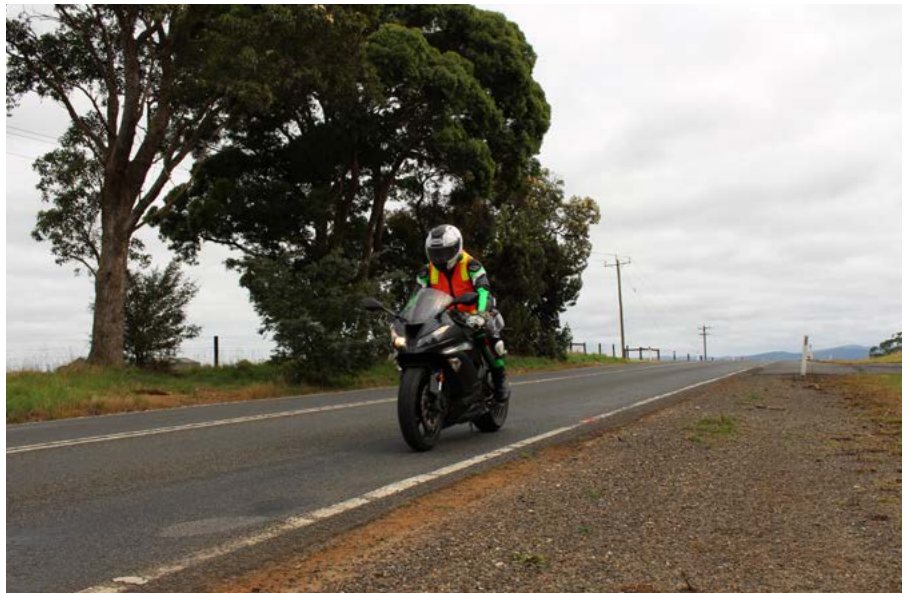
Unsealed shoulder with edge breaks makes recovery more difficult for motorcyclists.
