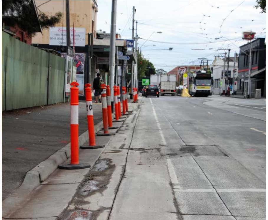
Rough surfaces in construction areas can result in a loss of traction for motorcyclists.
