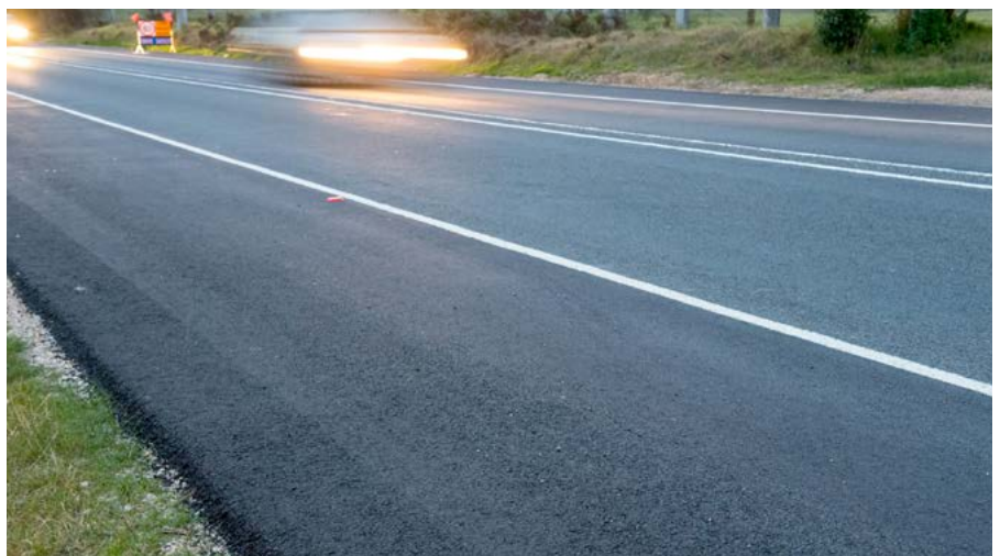
Sealed road shoulders provide a safe recovery area for all vehicles.
