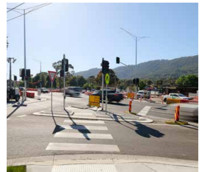
The new Montrose Road signalised pedestrian crossing is now operating.
