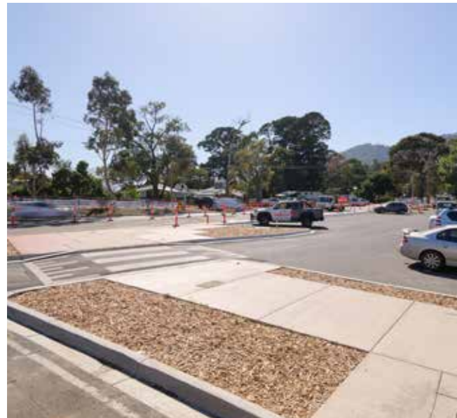
New angle parking and a raised pedestrian crossing at the Mount Dandenong Tourist Road shopping strip.
