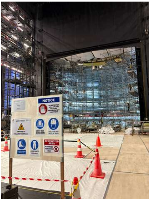
Upgrading works at the Esplanade Theatre in 2025.
