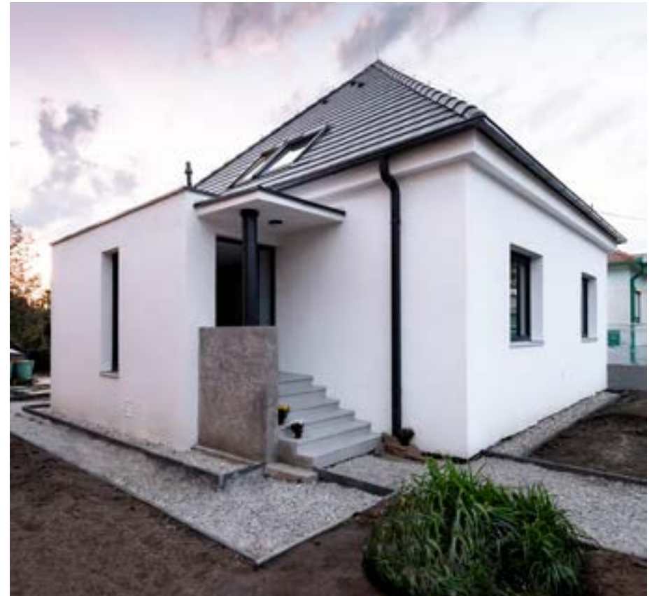
The home after renovation
