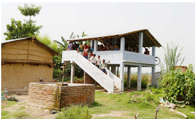
Evacuation platform and safe water source in Daulatpur, Karnali, Nepal
