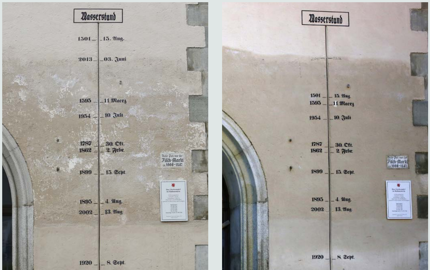
The photo on the left was taken in April 2014 and shows the level of flooding including the high-water mark from June 2013. The photo on the right, taken in June 2013 right after the floods, shows levels prior to when they were 'adjusted.' After reviewing history records and recalibrating various gauge levels, the 1501 flood still remains the worst in Passau's recorded history. Could the next flood top recorded levels? (See also text on opposite page).
