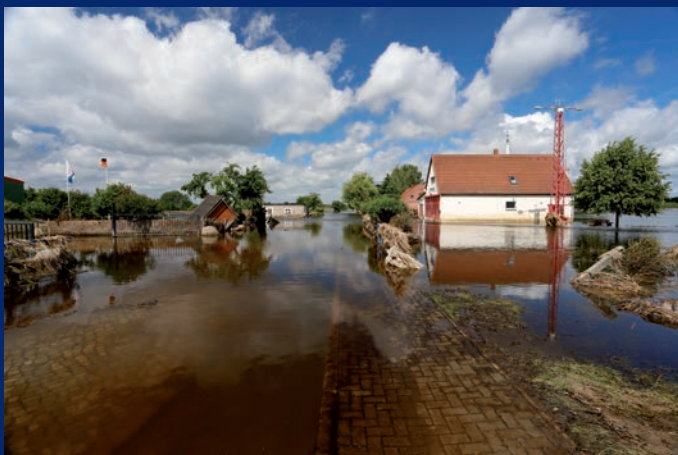
Cover photo comparison: The location affected by the Elbe levee breach in June 2013 and the same location revisited in April 2014.
