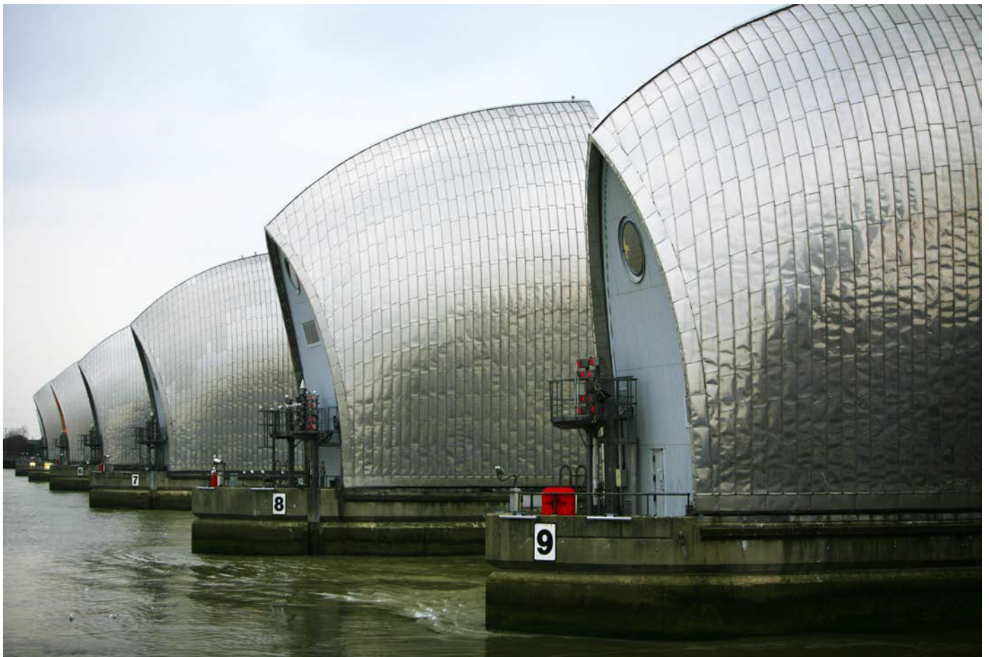
The Thames Barrier's gates can open and close to protect the Greater London area from storm surges of the North Sea.
