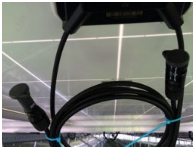
Example of a PV modules with unmatted connectors with protective caps (Picture/Illustration of Stäubli, Switzerland)
