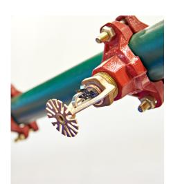
Inspect and hydrostatically test all water services (including fire sprinklers) and waste lines before charging and closing up walls and before installing ceilings and floors.
