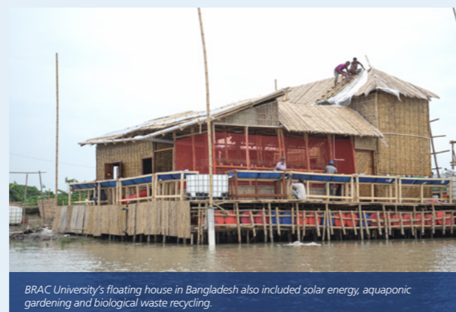
Retrofitting houses so that they float in a flood helps people stay in their homes and carry on their lives. With University of Waterloo in Vietnam.
